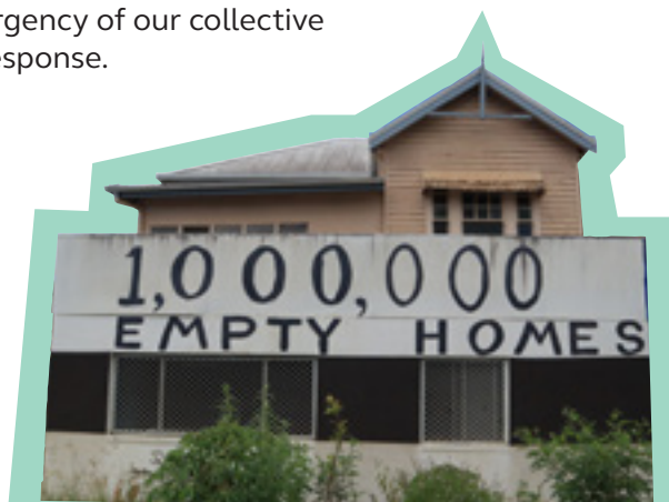
Graffiti on a house in North Lismore, after the devastating Northern Rivers region flooding.
